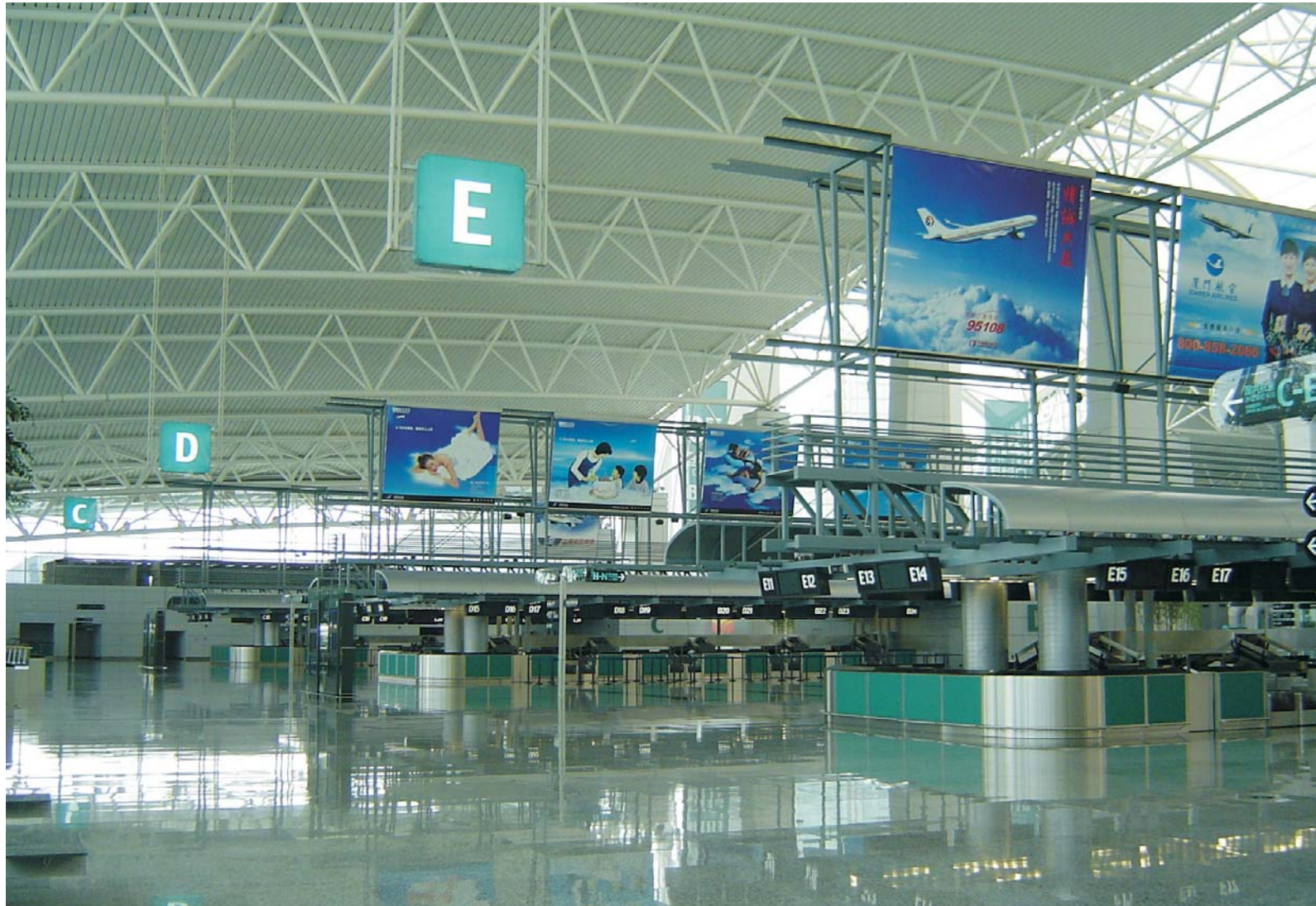
11 Check-in island canopies; powder coated Mild steel, with Aluminium cladding
