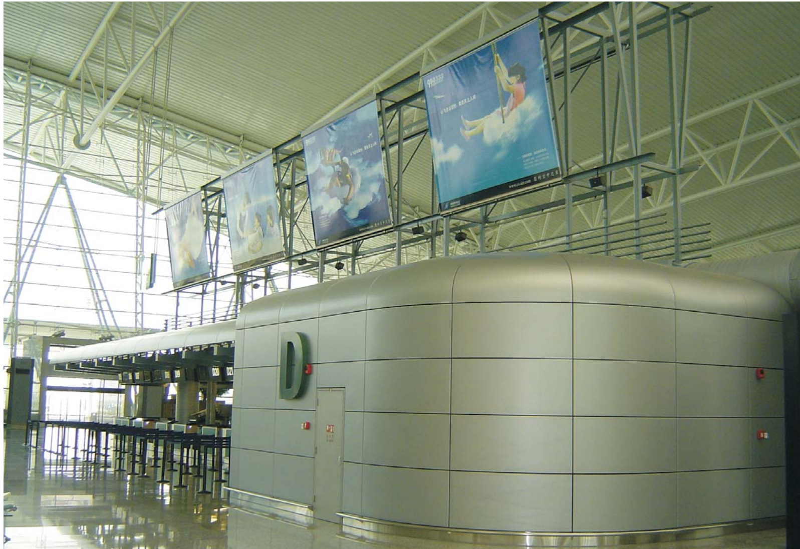
Guangzhou-Check-in island office module; Aluminium 3 D curved cladding
