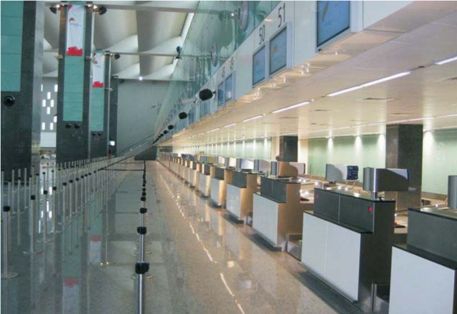
Check-in row, Mild+stainless steel counters with composite stone top
